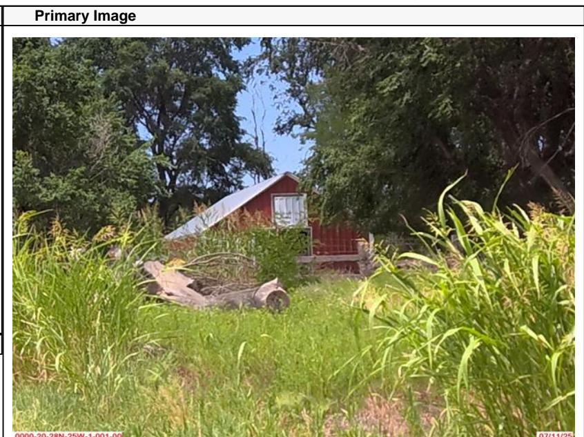
0000-20-28N-25W-1-001-001 07/11/25 RED METAL SHED 7/15/2025
