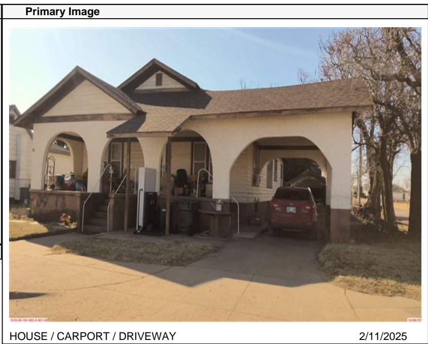
HOUSE / CARPORT / DRIVEWAY 2/11/2025
