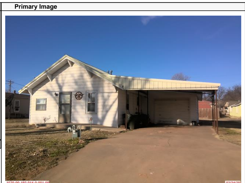
1070-00-192-014-0-001-00 02/24/25 HOUSE / CARPORT / ATTACHED GARAGE & DRIVEWAY 2/24/2025
