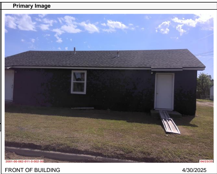
FRONT OF BUILDING 4/30/2025
