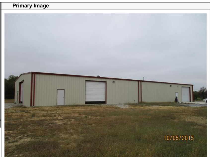
NEW ADDITION TO EXISTING SHOP 10/5/2015
