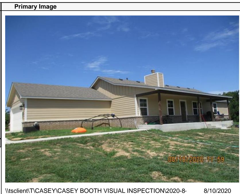
\\tsclient\TCASEY\CASEY BOOTH VISUAL INSPECTION\2020-8- 8/10/2020
