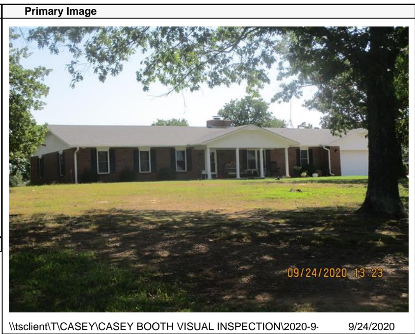
\\tsclient\TCASEY\CASEY BOOTH VISUAL INSPECTION\2020-9- 9/24/2020
