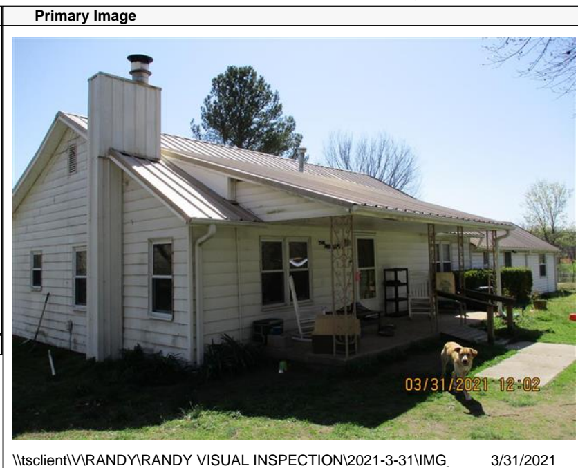
\\tsclient\VRANDY\RANDY VISUAL INSPECTION\2021-3-31\IMG_ 3/31/2021
