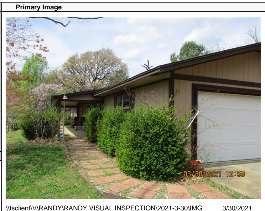
\\tsclient\VRANDY\RANDY VISUAL INSPECTION\2021-3-30\IMG_ 3/30/2021
