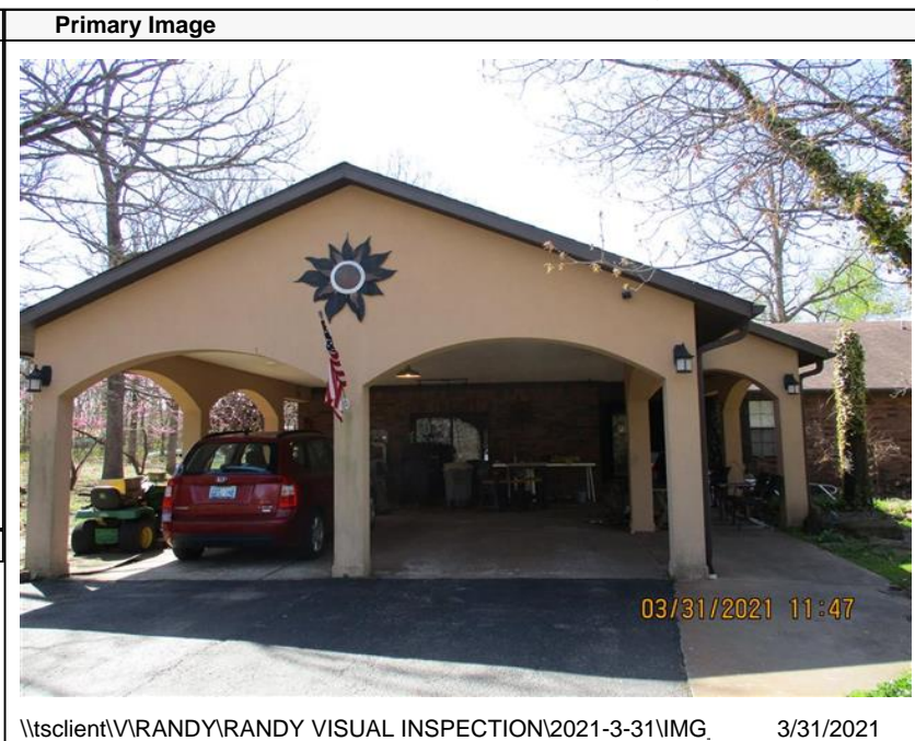
\\tsclient\VRANDY\RANDY VISUAL INSPECTION\2021-3-31\IMG_ 3/31/2021
