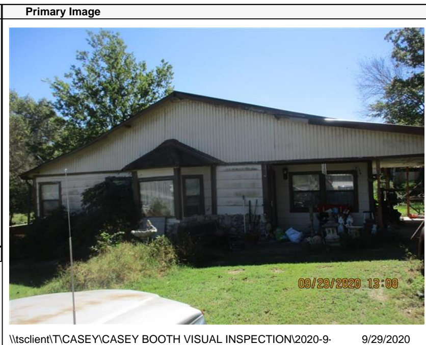
\\tsclient\TCASEY\CASEY BOOTH VISUAL INSPECTION\2020-9- 9/29/2020
