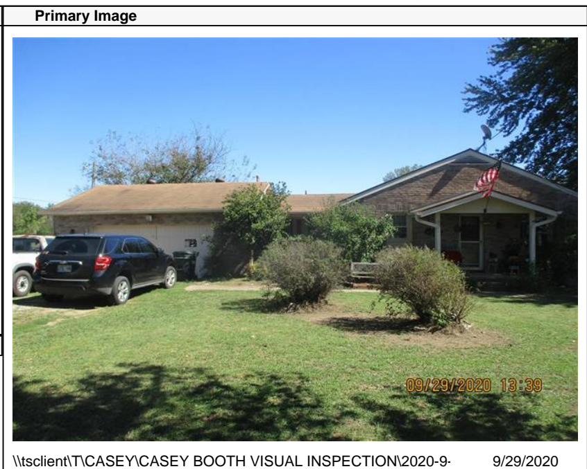
\\tsclient\TCASEY\CASEY BOOTH VISUAL INSPECTION\2020-9- 9/29/2020
