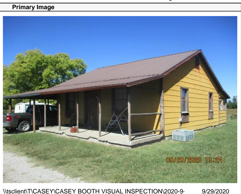
\\tsclient\TCASEY\CASEY BOOTH VISUAL INSPECTION\2020-9- 9/29/2020
