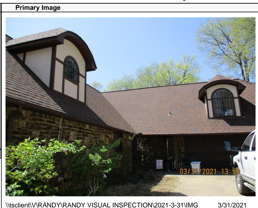
\\tsclient\VRANDY\RANDY VISUAL INSPECTION\2021-3-31\IMG_ 3/31/2021
