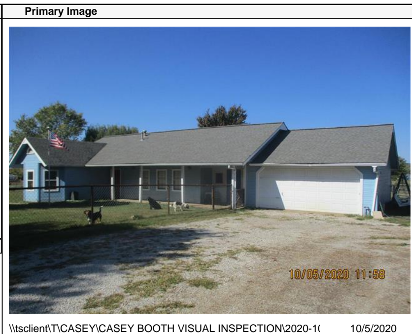
\\tsclient\TCASEY\CASEY BOOTH VISUAL INSPECTION\2020-1( 10/5/2020
