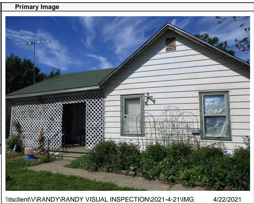
\\tsclient\VRANDY\RANDY VISUAL INSPECTION\2021-4-21\IMG_ 4/22/2021
