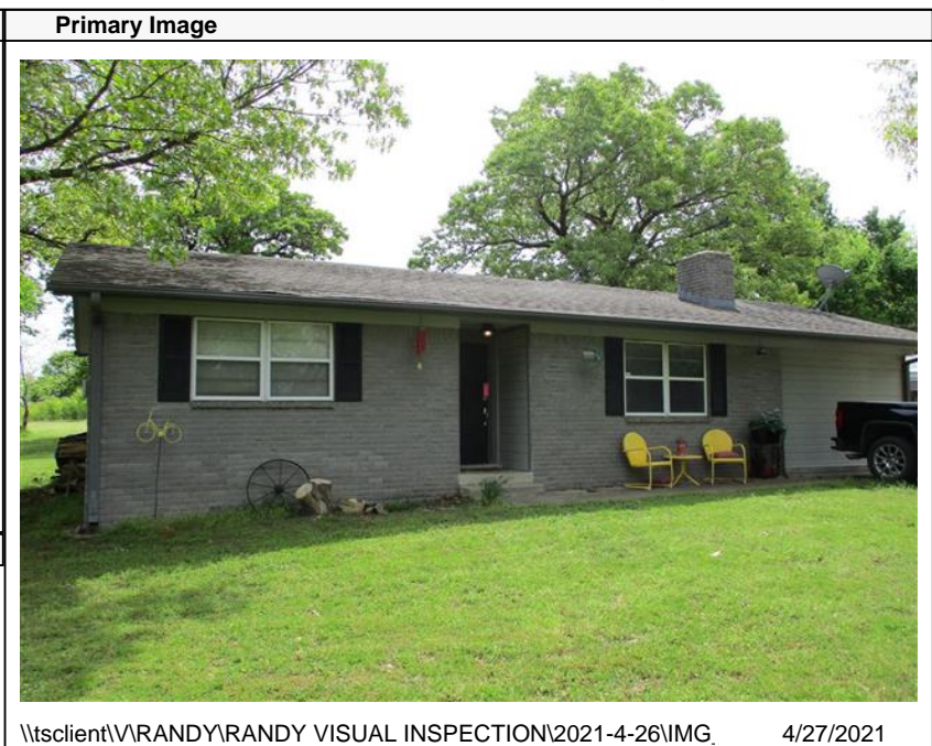
\\tsclient\VRANDY\RANDY VISUAL INSPECTION\2021-4-26\IMG_ 4/27/2021
