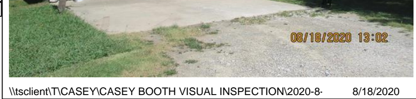
\\tsclient\TCASEY\CASEY BOOTH VISUAL INSPECTION\2020-8- 8/18/2020
