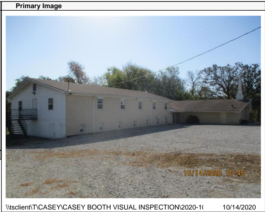
\\tsclient\TCASEY\CASEY BOOTH VISUAL INSPECTION\2020-1( 10/14/2020
