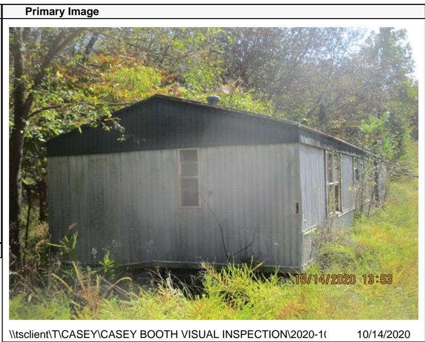
\\tsclient\TCASEY\CASEY BOOTH VISUAL INSPECTION\2020-1( 10/14/2020
