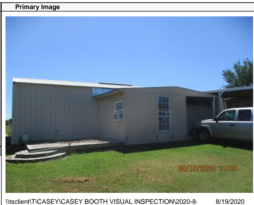
\\tsclient\TCASEY\CASEY BOOTH VISUAL INSPECTION\2020-8- 8/19/2020
