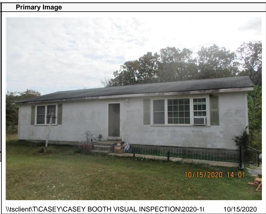
\\tsclient\TCASEY\CASEY BOOTH VISUAL INSPECTION\2020-1( 10/15/2020
