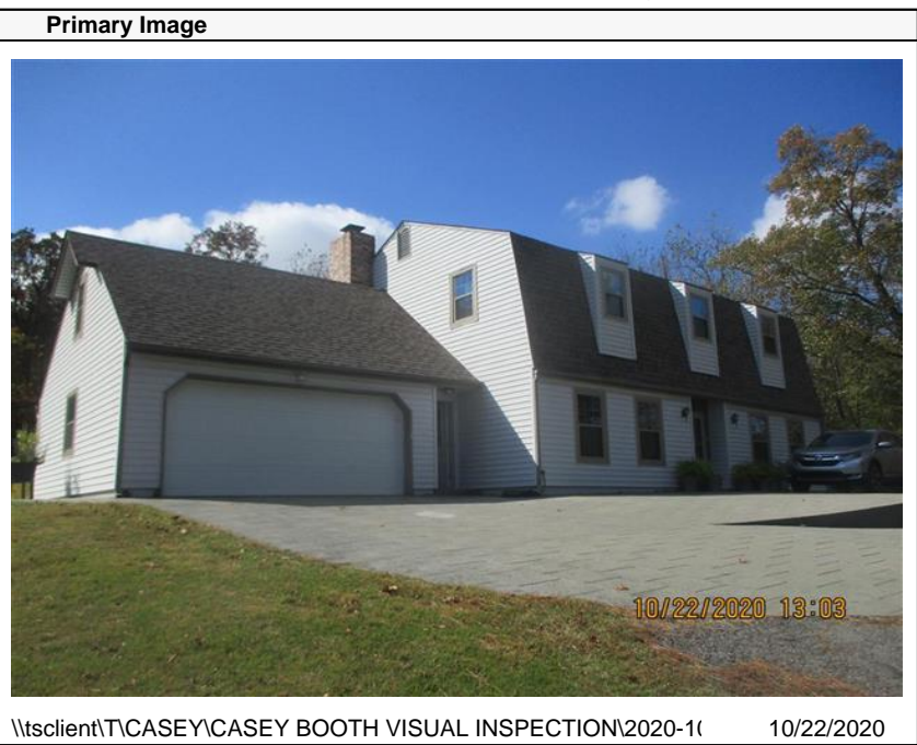
\\tsclient\TCASEY\CASEY BOOTH VISUAL INSPECTION\2020-1( 10/22/2020
