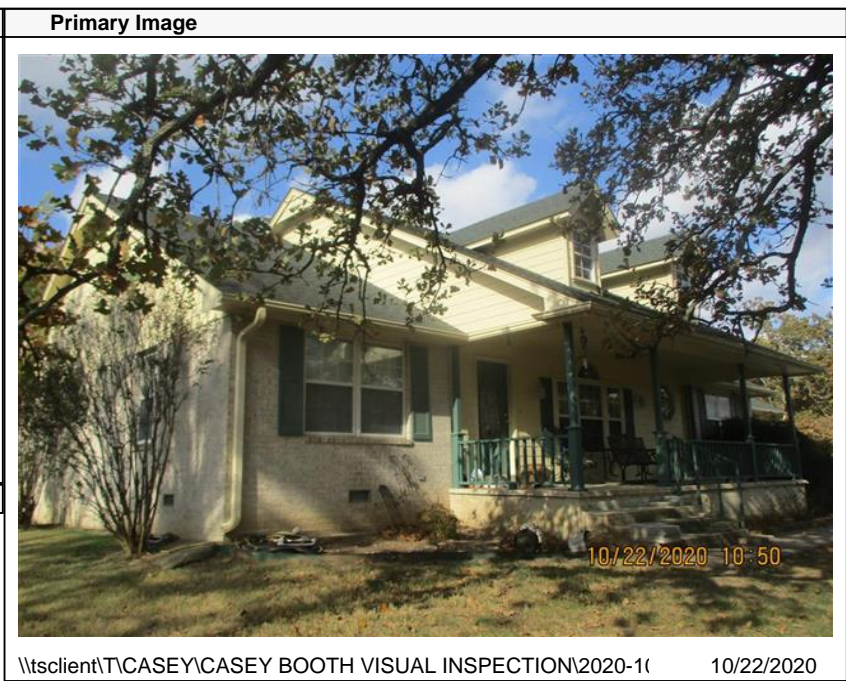
\\tsclient\TCASEY\CASEY BOOTH VISUAL INSPECTION\2020-1( 10/22/2020
