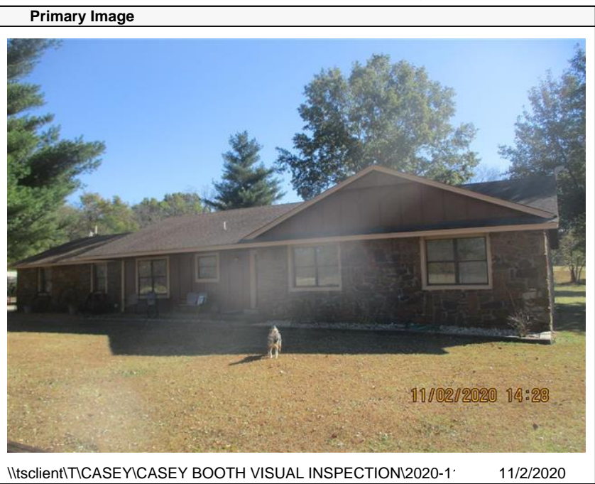
\\tsclient\TCASEY\CASEY BOOTH VISUAL INSPECTION\2020-1' 11/2/2020
