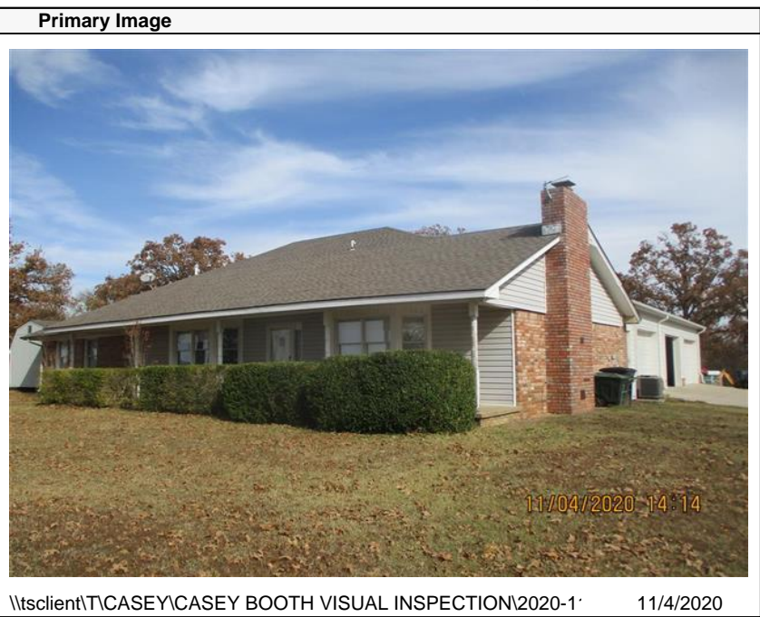
\\tsclient\TCASEY\CASEY BOOTH VISUAL INSPECTION\2020-1' 11/4/2020
