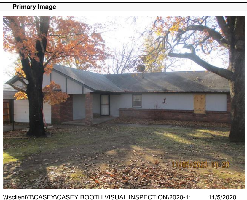
\\tsclient\TCASEY\CASEY BOOTH VISUAL INSPECTION\2020-1' 11/5/2020
