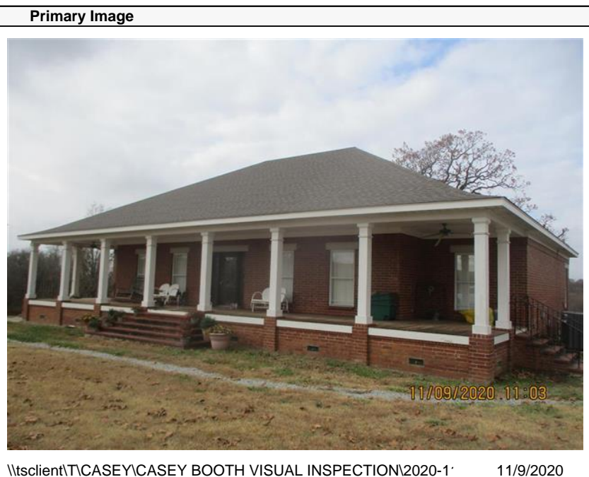
\\tsclient\TCASEY\CASEY BOOTH VISUAL INSPECTION\2020-1' 11/9/2020
