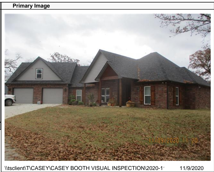
\\tsclient\TCASEY\CASEY BOOTH VISUAL INSPECTION\2020-1\ 11/9/2020
