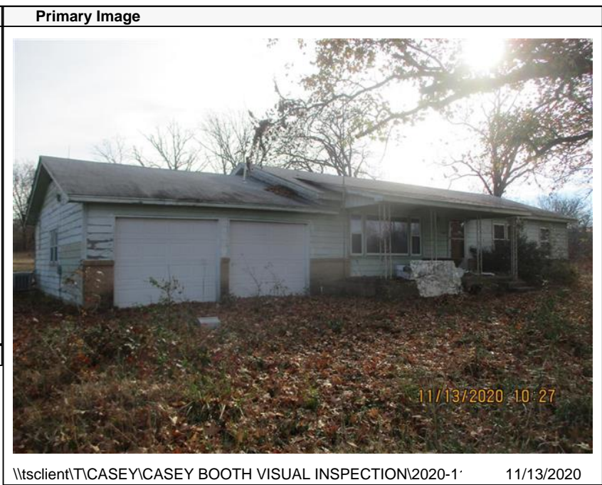
\\tsclient\TCASEY\CASEY BOOTH VISUAL INSPECTION\2020-1\ 11/13/2020
