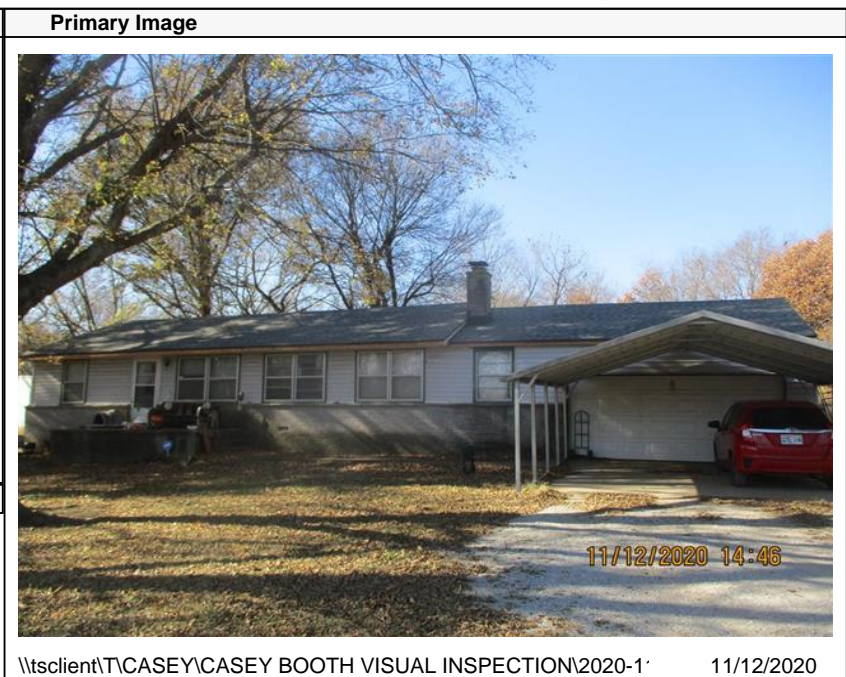
\\tsclient\TCASEY\CASEY BOOTH VISUAL INSPECTION\2020-1' 11/12/2020
