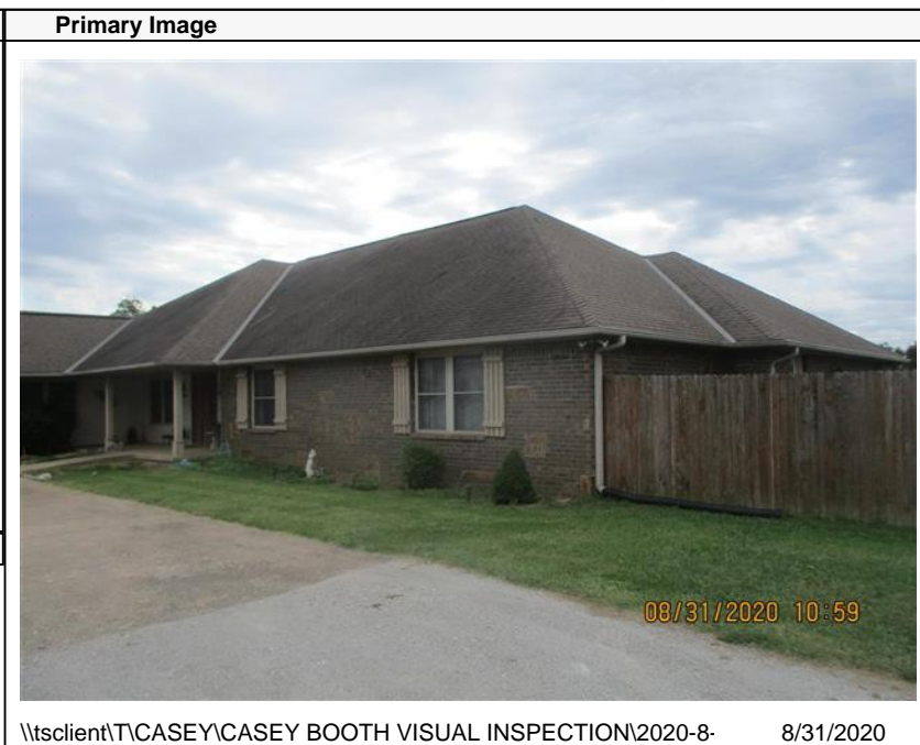
\\tsclient\TCASEY\CASEY BOOTH VISUAL INSPECTION\2020-8- 8/31/2020
