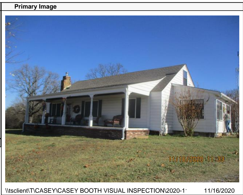
\\tsclient\TCASEY\CASEY BOOTH VISUAL INSPECTION\2020-1' 11/16/2020
