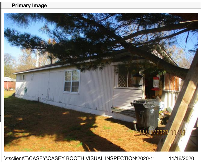
\\tsclient\TCASEY\CASEY BOOTH VISUAL INSPECTION\2020-1' 11/16/2020
