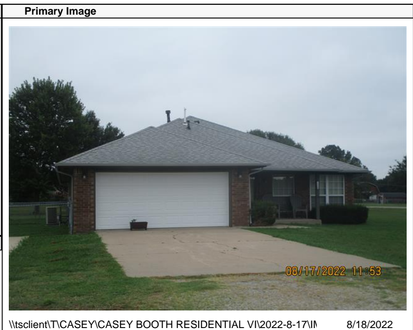
\\tsclient\TCASEY\CASEY BOOTH RESIDENTIAL VI\2022-8-17\ 8/18/2022
