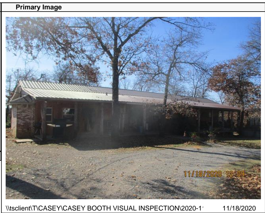
\\tsclient\TCASEY\CASEY BOOTH VISUAL INSPECTION\2020-1' 11/18/2020
