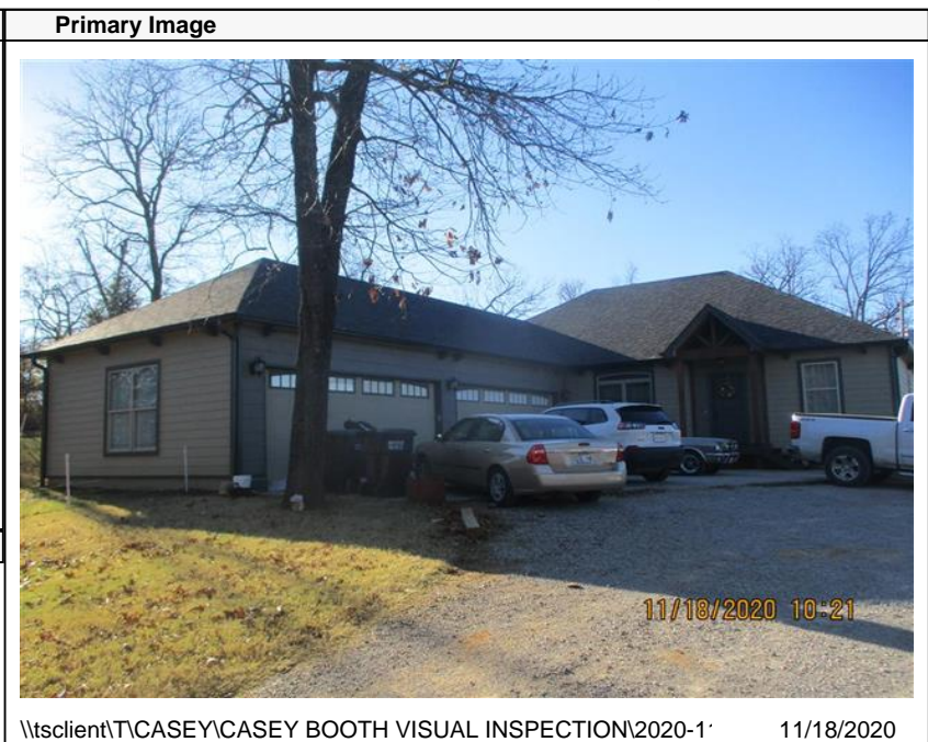
\\tsclient\TCASEY\CASEY BOOTH VISUAL INSPECTION\2020-1' 11/18/2020
