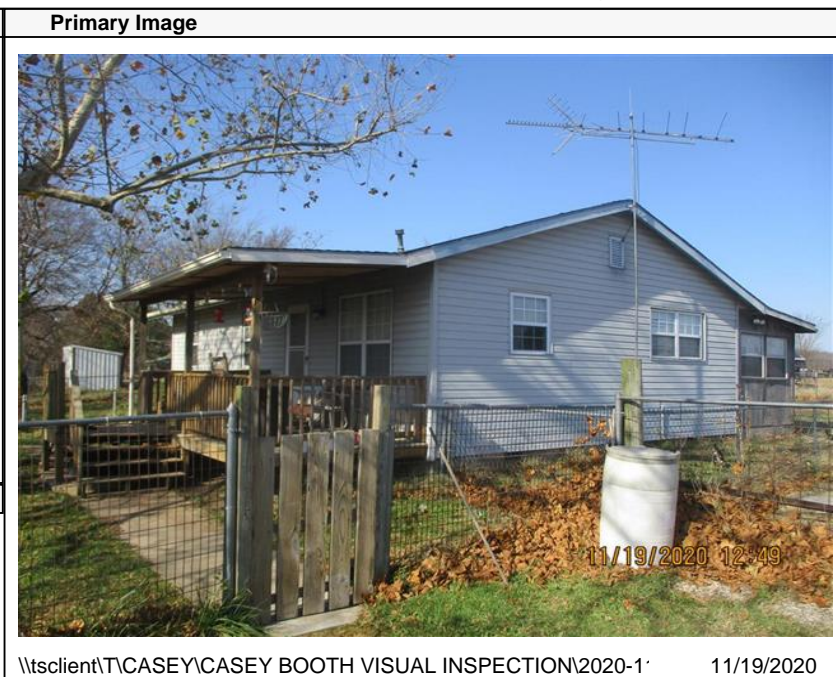
\\tsclient\TCASEY\CASEY BOOTH VISUAL INSPECTION\2020-1' 11/19/2020
