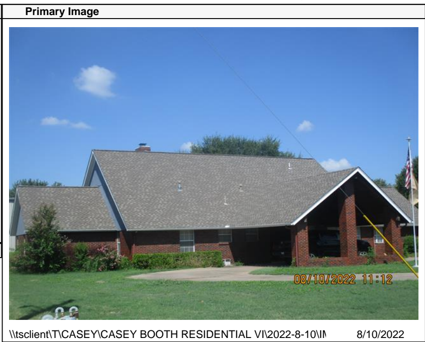
\\tsclient\TCASEY\CASEY BOOTH RESIDENTIAL VI\2022-8-10\ 8/10/2022
