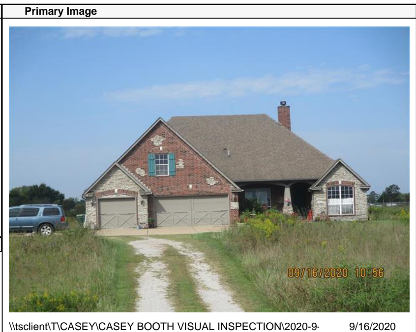
\\tsclient\TCASEY\CASEY BOOTH VISUAL INSPECTION\2020-9- 9/16/2020
