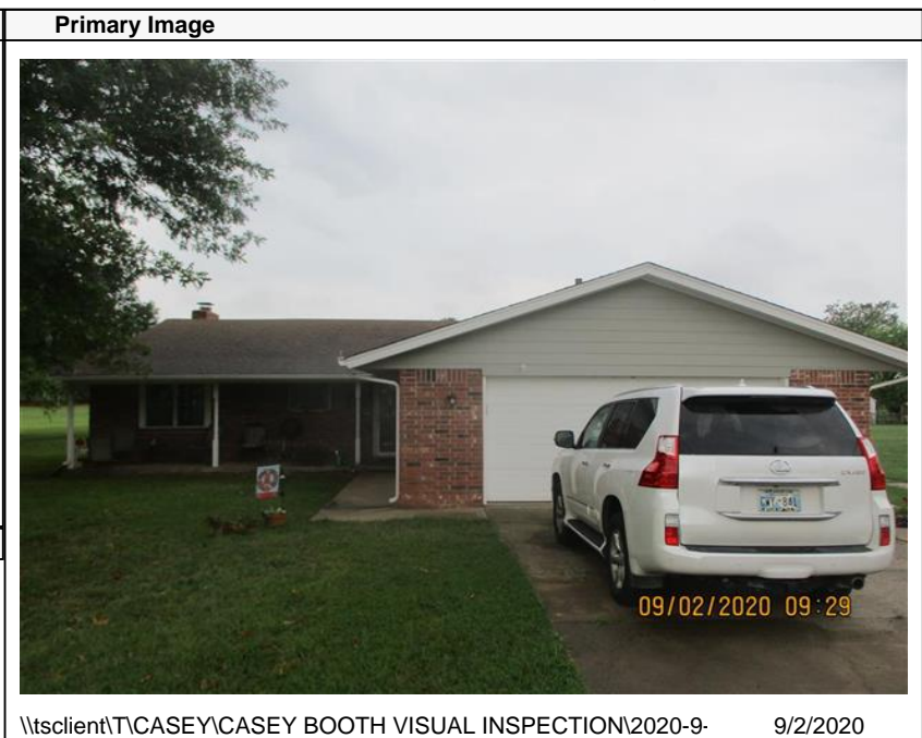
\\tsclient\TCASEY\CASEY BOOTH VISUAL INSPECTION\2020-9- 9/2/2020
