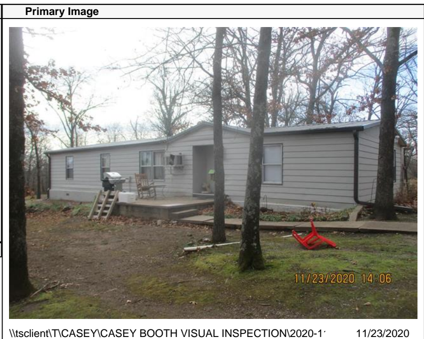
\\tsclient\TCASEY\CASEY BOOTH VISUAL INSPECTION\2020-1' 11/23/2020
