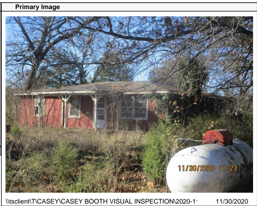
\\tsclient\TCASEY\CASEY BOOTH VISUAL INSPECTION\2020-1' 11/30/2020
