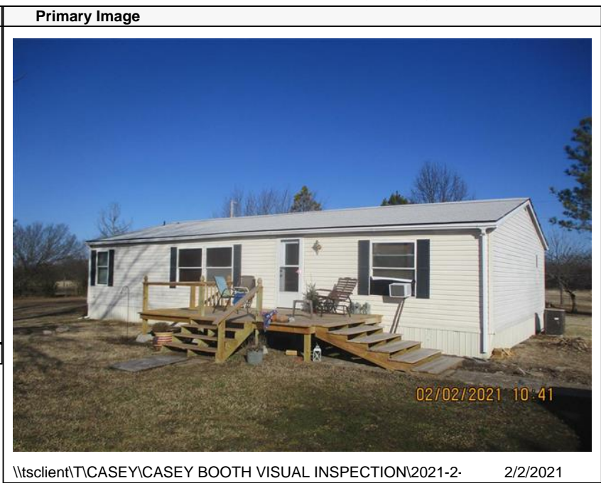
\\tsclient\TCASEY\CASEY BOOTH VISUAL INSPECTION\2021-2- 2/2/2021
