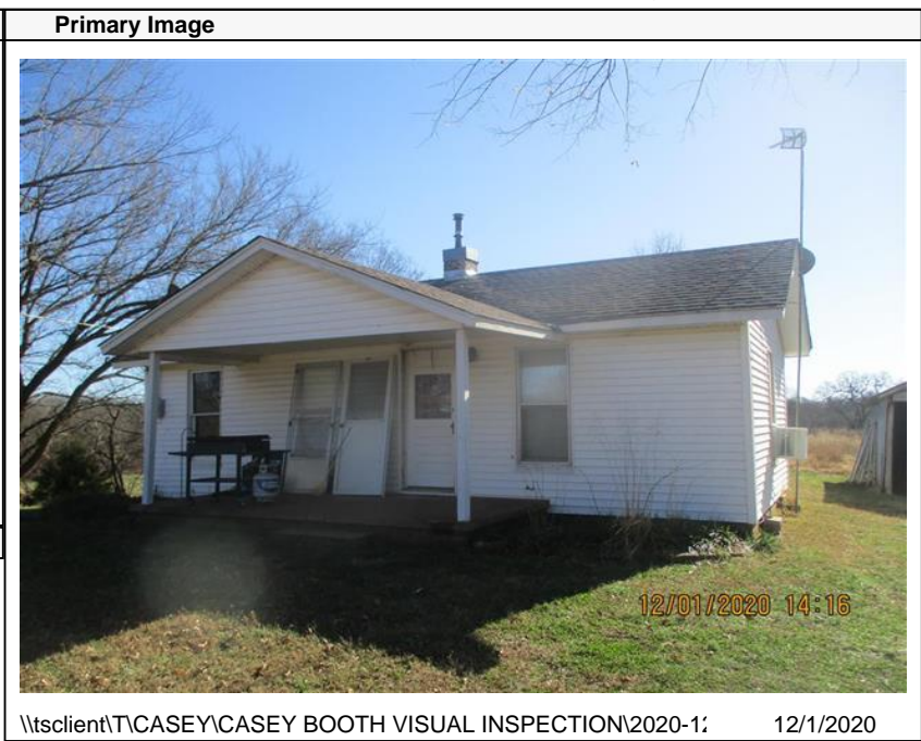
\\tsclient\TCASEY\CASEY BOOTH VISUAL INSPECTION\2020-1; 12/1/2020
