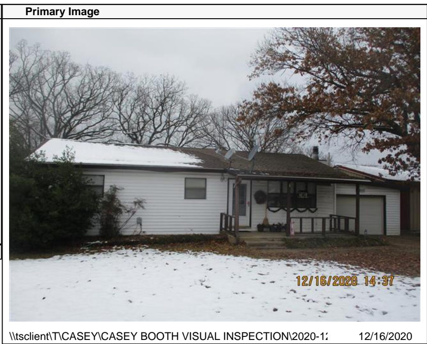
\\tsclient\TCASEY\CASEY BOOTH VISUAL INSPECTION\2020-1; 12/16/2020
