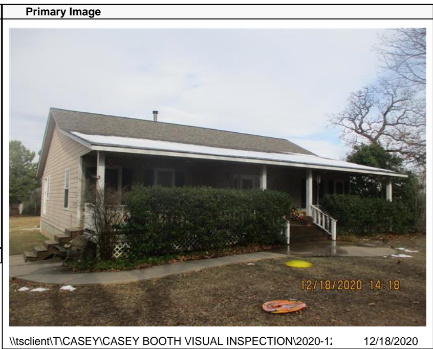
\\tsclient\TCASEY\CASEY BOOTH VISUAL INSPECTION\2020-1; 12/18/2020
