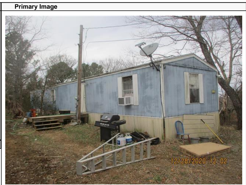
\\tsclient\T\CASEY\CASEY BOOTH VISUAL INSPECTION\2020-1; 12/28/2020
