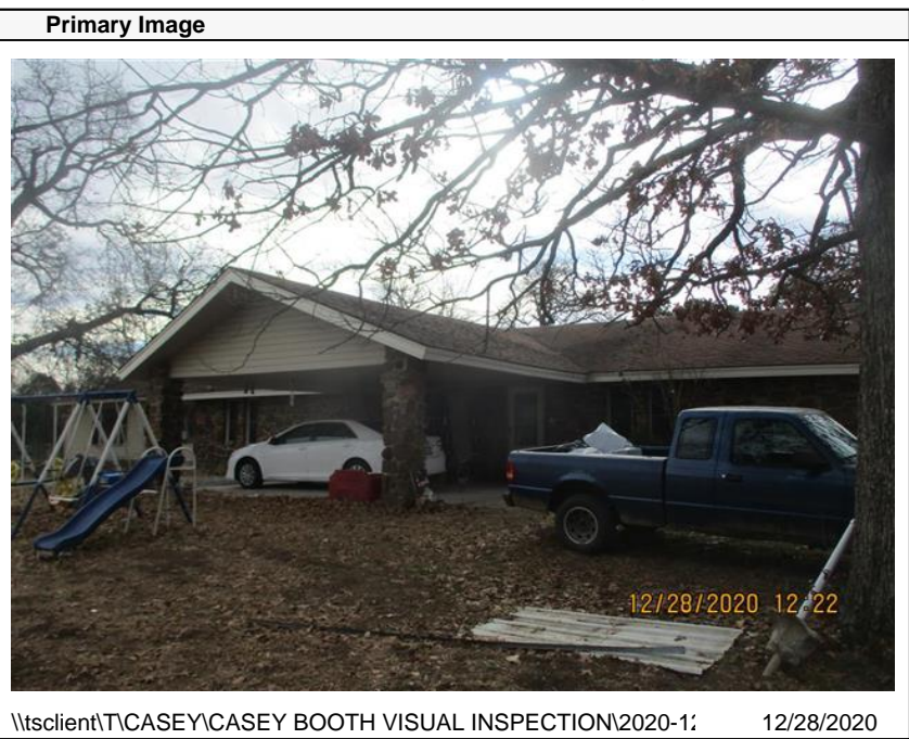
\\tsclient\TCASEY\CASEY BOOTH VISUAL INSPECTION\2020-1; 12/28/2020
