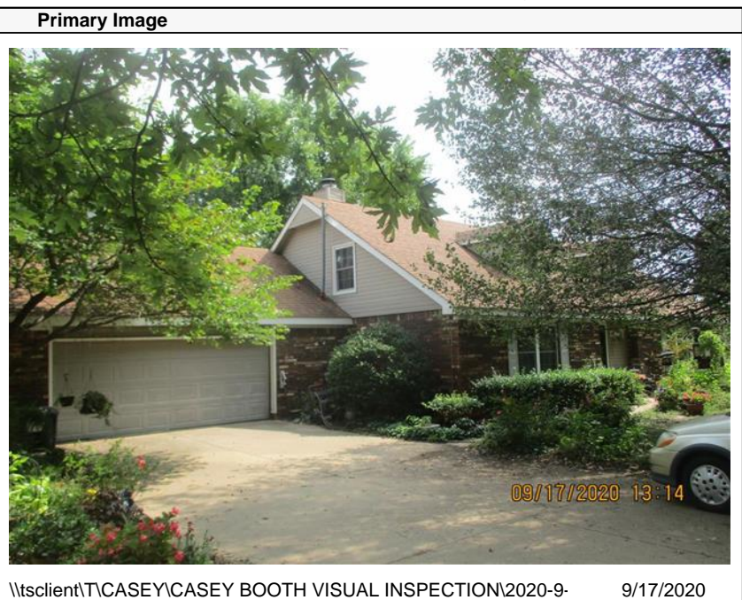
\\tsclient\TCASEY\CASEY BOOTH VISUAL INSPECTION\2020-9- 9/17/2020
